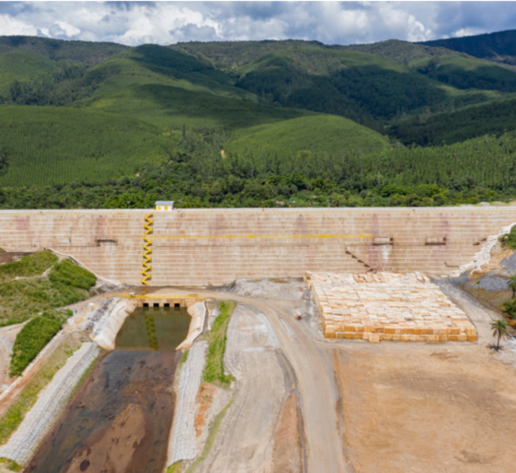
Implementation of the downstream containment (backup dam) of the Sul Superior Dam, in Barão de Cocais.
