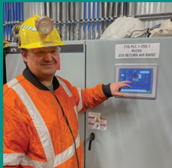
Powering up the new 350 Return Air Raise for the first time.
