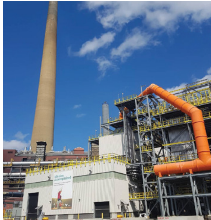
Smelter at Copper Cliff.
