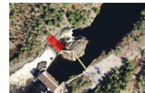
An aerial view of the Nairn Falls generation station.
