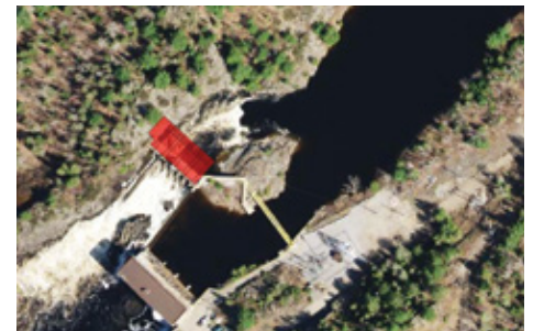
An aerial view of the Nairn Falls generation station.
