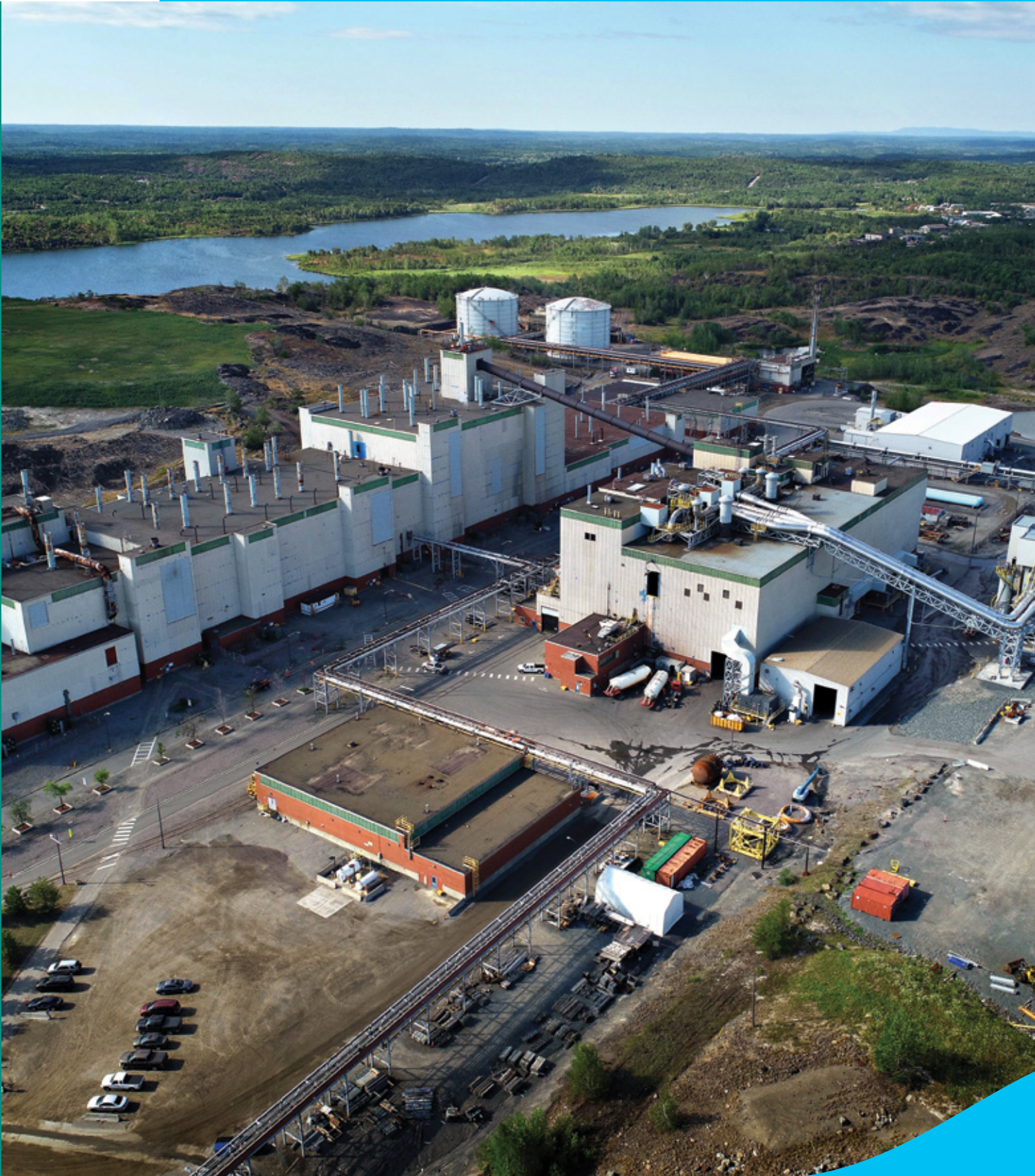
Aerial view of Copper Cliff Nickel Refinery.
