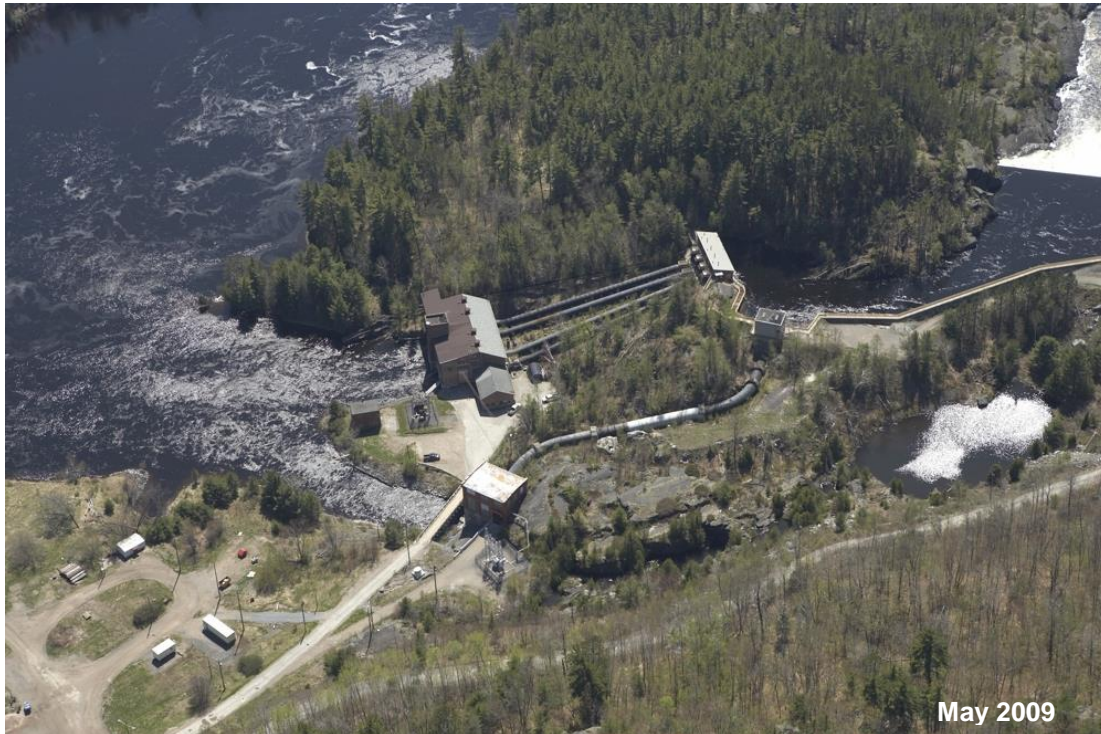
High Falls No.1 / No.2 and Big Eddy Dams and Generating Plants
