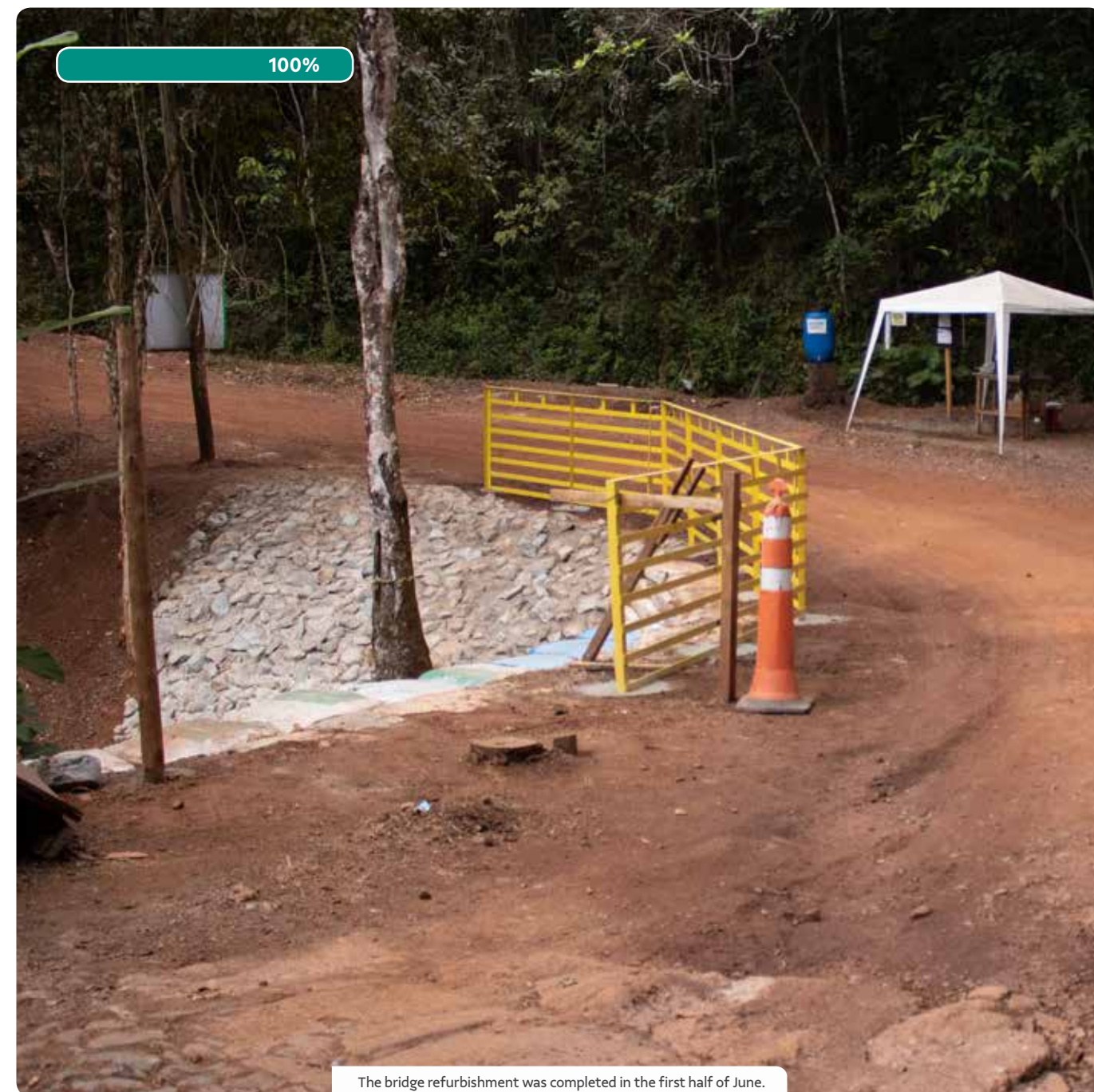
The bridge refurbishment was completed in the first half of June.
