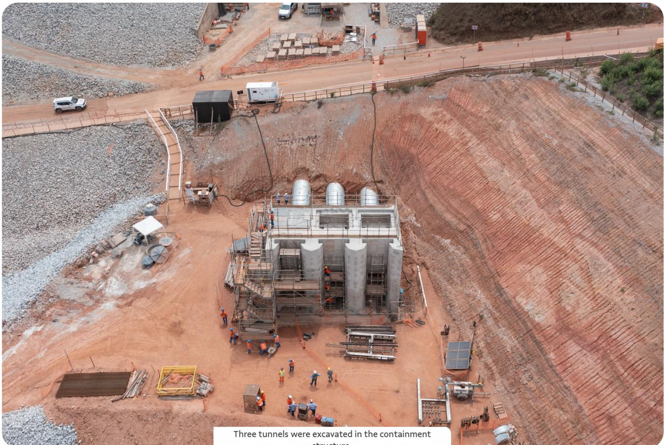
Three tunnels were excavated in the containment structure.
