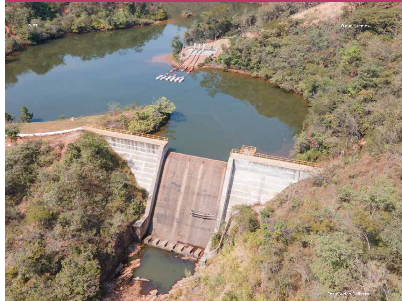
Intake and pipeline at the Cambimbe dam
