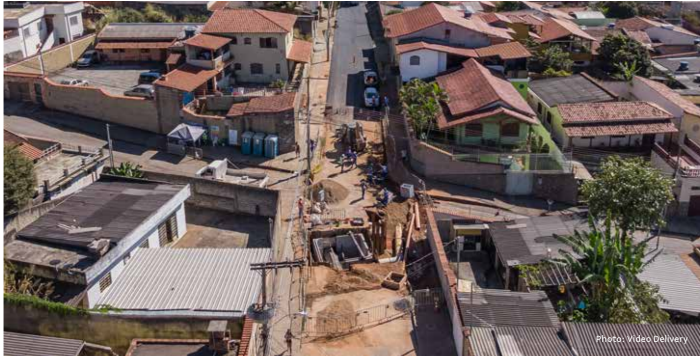
Installation works for the Carlos Prates water pipeline, in Belo Horizonte
