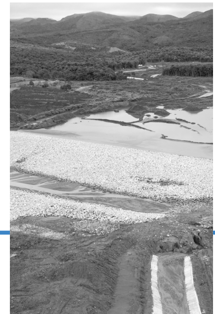
Hydraulic Barrier 1 (BH1). Photo: Vale Archive.
