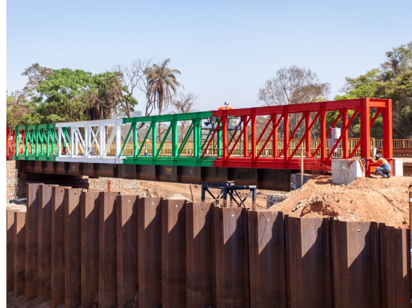
Sheet Pile- General View. Photo: Vale Archive.
