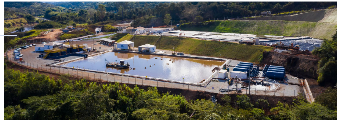
River Water Treatment Station (ETAF), in Brumadinho (MG). Photo: Vale Archive.
