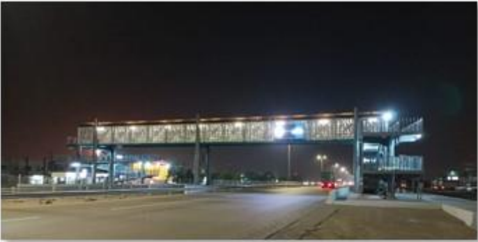
Overpass Pedestrian Construction at Liwa
