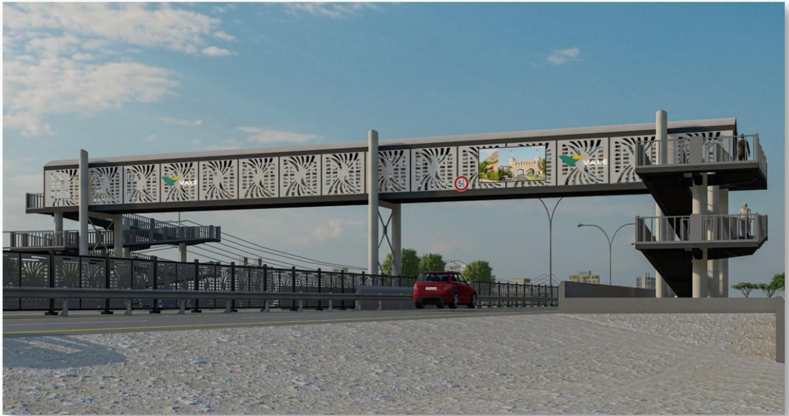
Overpass Pedestrian Construction at Liwa
