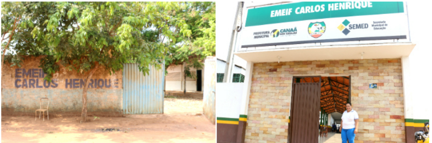
Carlos Henrique Municipal School in Canaã dos Carajás, before and after the renovation
