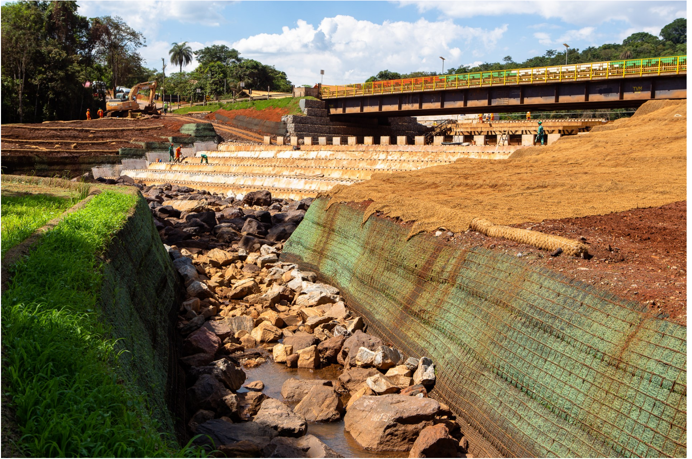
Stream channel was re-created with rocks at the bottom and walls of biomantle (revegetation).
