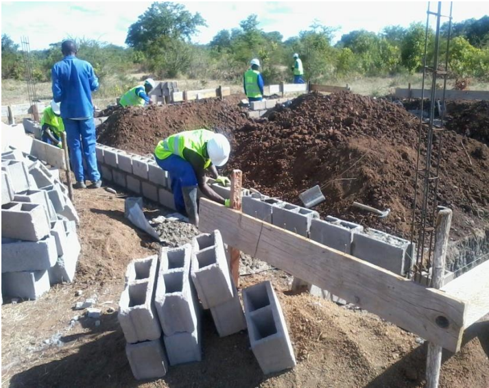
Construction of Mr. Raúl Chauma house.
