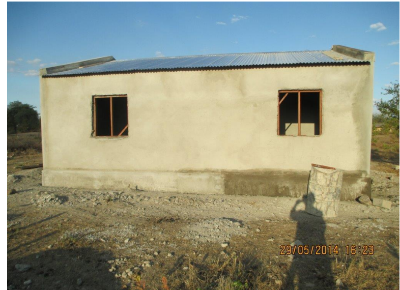
House under construction at Nhamitsatse community.
